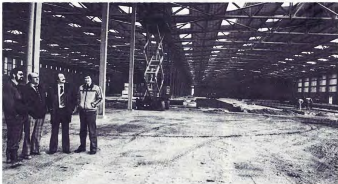
A section of the massive new Hotpoint factory at Bodelwyddan. In the picture we see, from left to right: Messrs. Gary Purchase (Hotpoint), Tommy Davies (foreman electrician), John Stobbs (Hotpoint) and Graham Monks.
